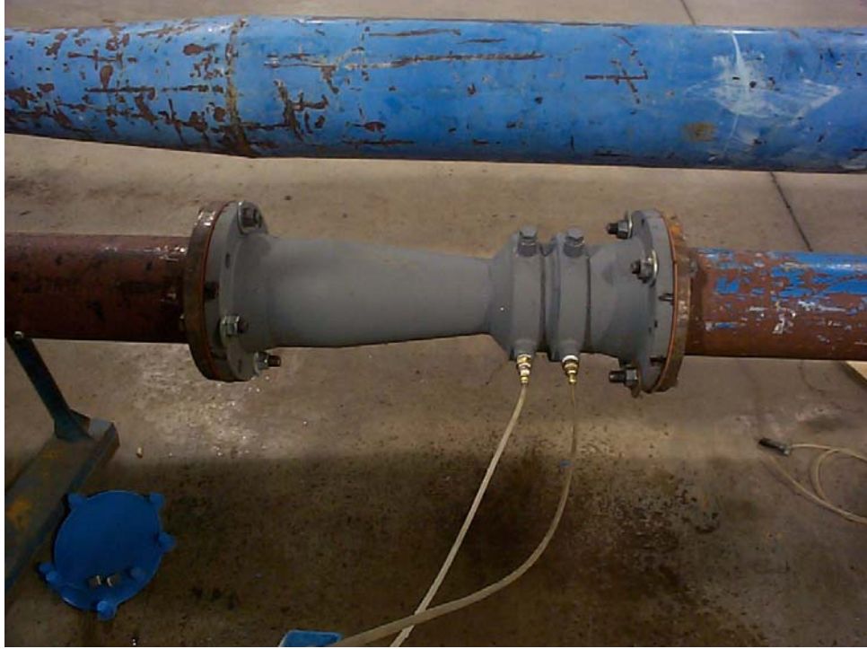
Figure 2. Installation of the 6-inch flow meter.
