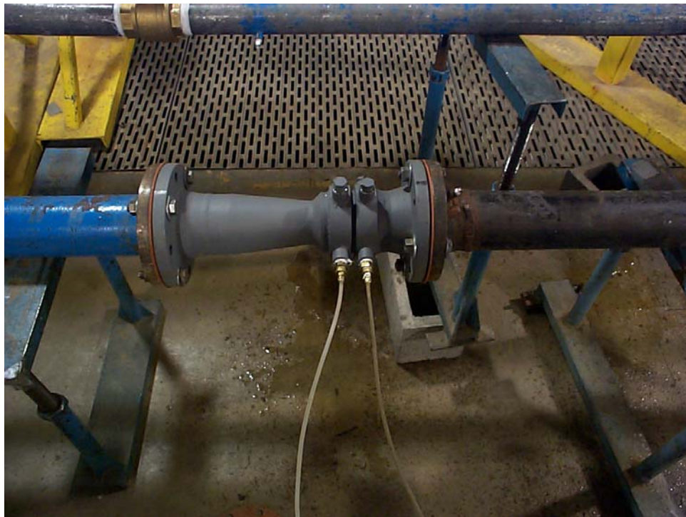
Figure 1. Installation of the 4-inch flow meter.
