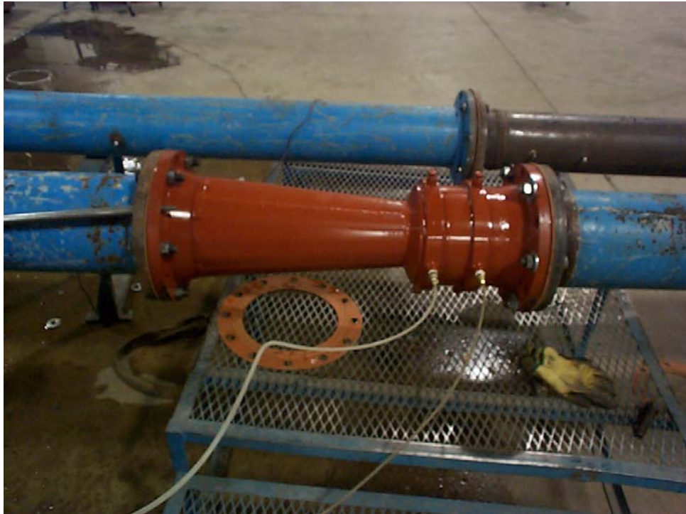
Figure 3. Installation of the 10-inch flow meter.
